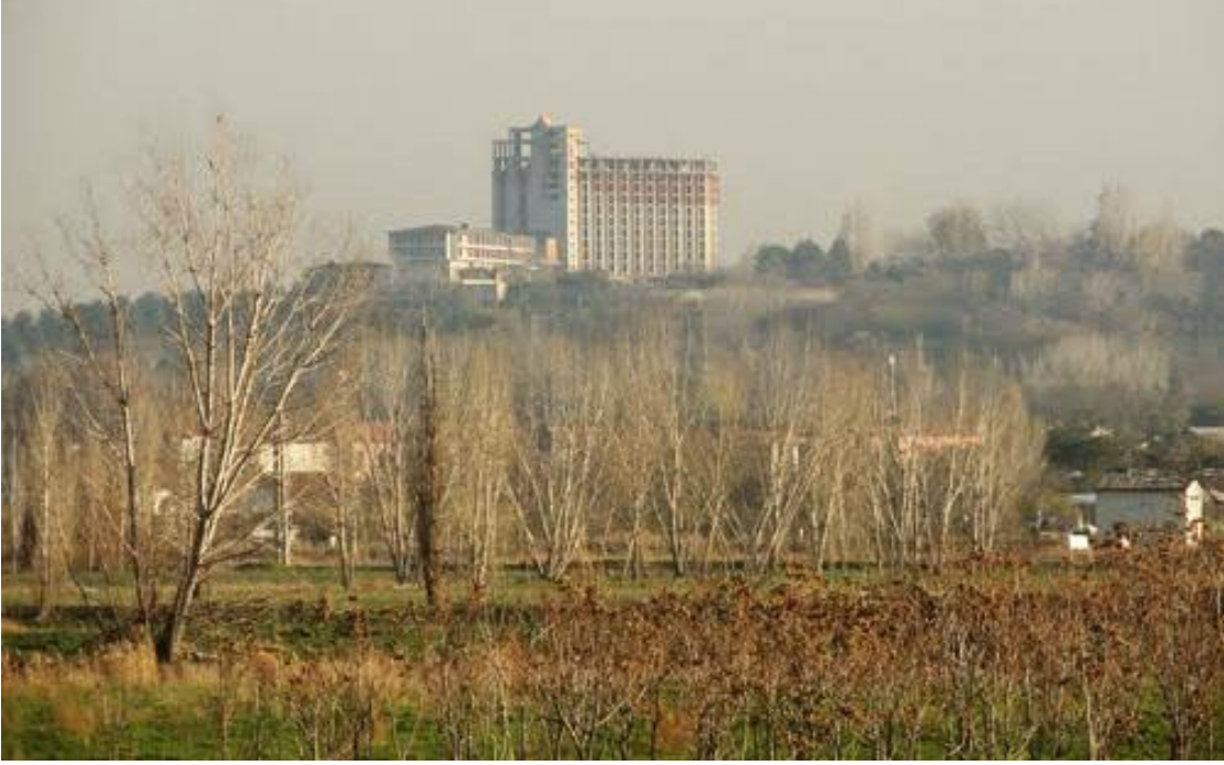
| Marmara Hotel on the silhouette of AOÇ land, Gazi Settlement
