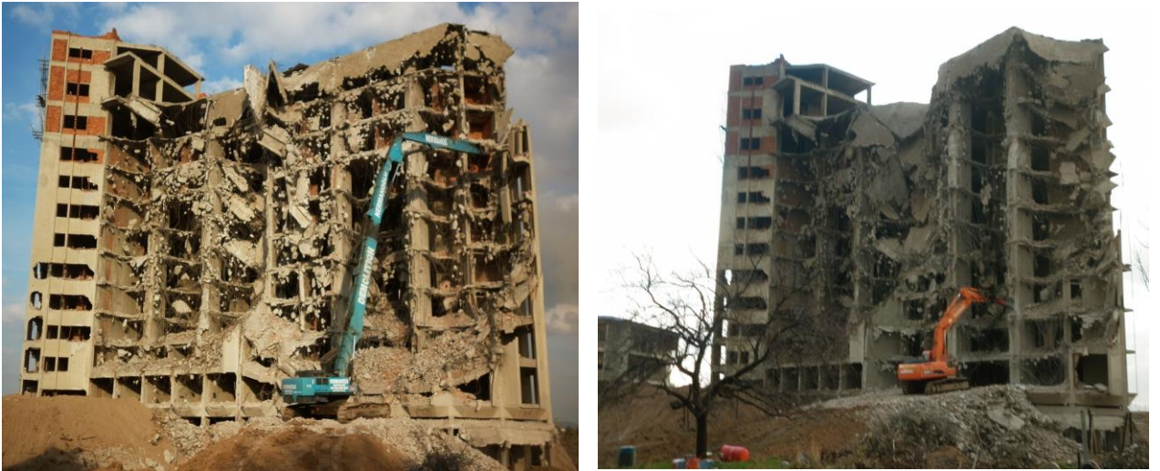
| Demolishing Process of the Hotel
