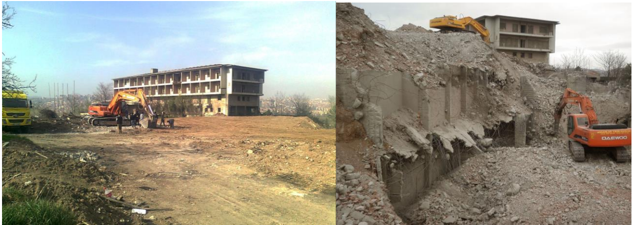
| The Initial Marmara Hotel Building on the Demolishing Process
