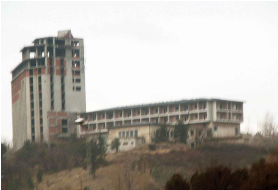
| A Closer Look to the Rough Construction of Marmara Hotel on AOÇ land, 2
